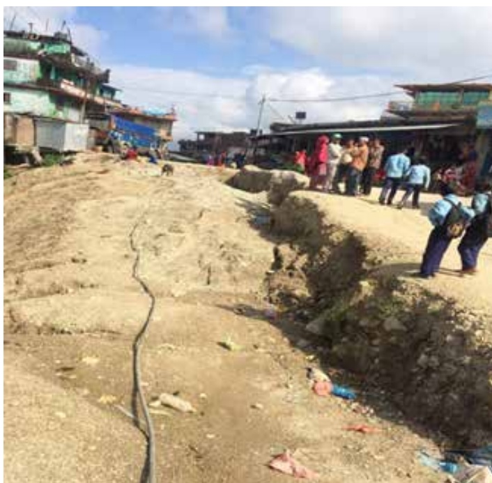
Pic 2: Highway that runs through Kapurkot Municipality has a major creeping landslide. Seen here in a differential settlement along the highway. The cracks along the road are reported to be increasing every year. Pic: Survey Team.
